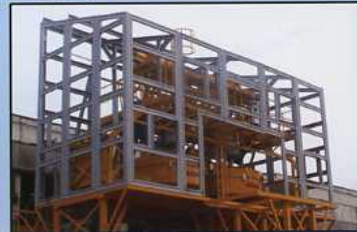
Metal construction under covering, special "sigma" profiles, bolt connections.
